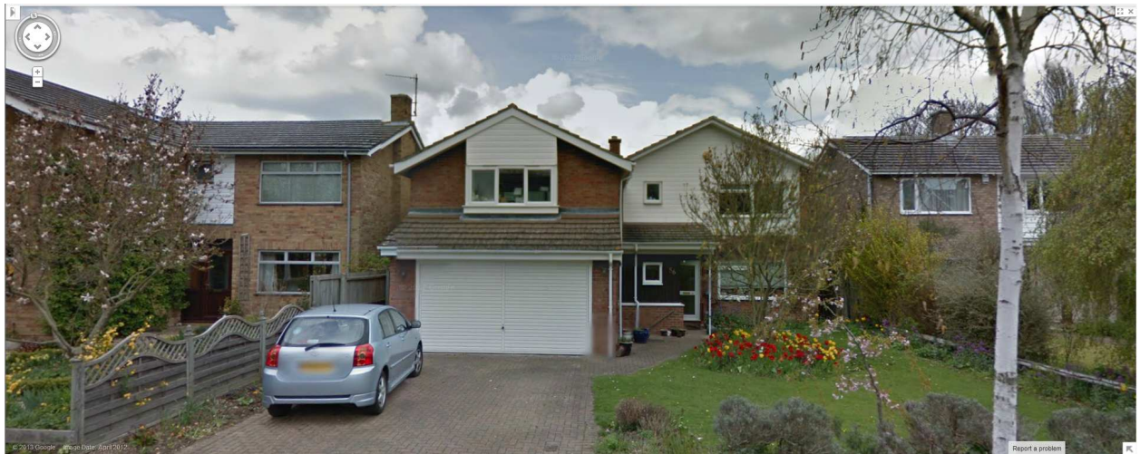
View looking east from Gough Way
